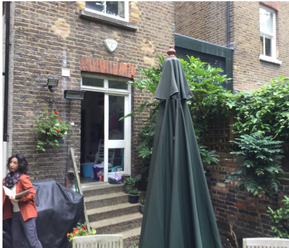
Rear of Existing Closet Wing
