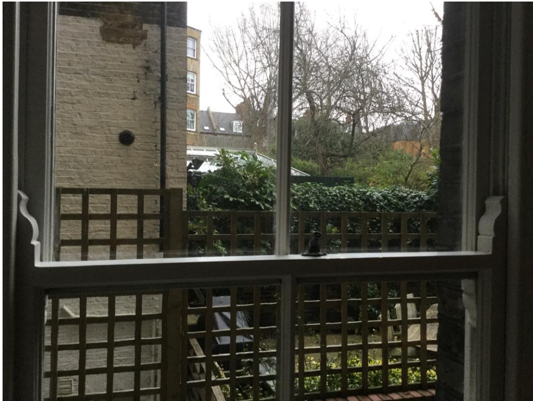
View of rear of 5 Maida Avenue from window in flat in Douglas House
